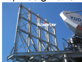
Reflection Reduction at 6.3GHz Antenna
